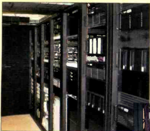
Ten racks face the distribution wall. Most of these racks were prewired by RDA Systems before being shipped to Omaha.
