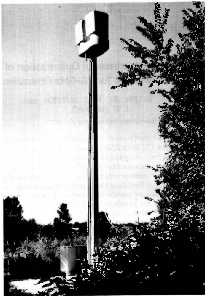
Fig. 1—DR 18A repeater site located in Methuen, Massachusetts.
