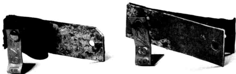
Fig. 14—Heavier corrosion at the interface of the polychloroprene-to-aluminum bond than on the exposed side of the metal strip.
