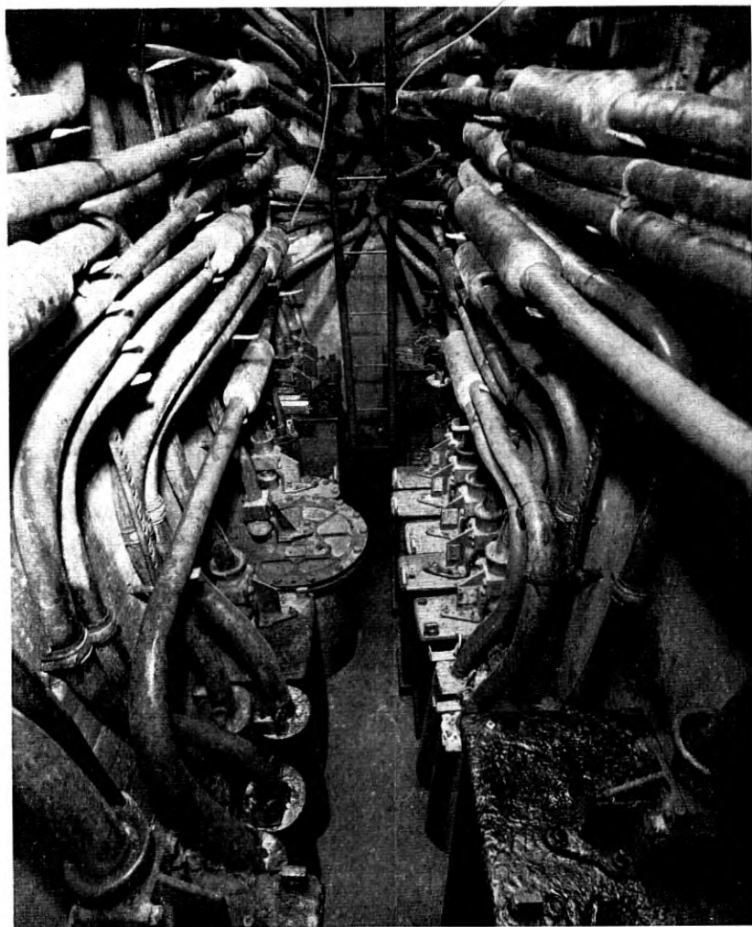
Fig. 28B—Other end of vault in Fig. 28A.
