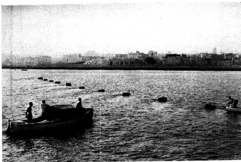
Fig. 16—Havana landing site.
