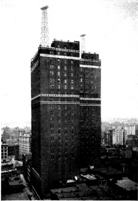
Fig. 17—Long distance telephone building, New York City
