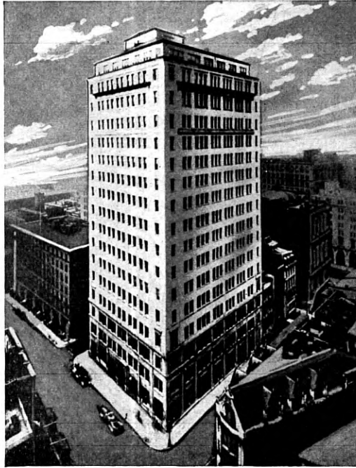
Fig. 15—Bowling Green telephone building, New York City
