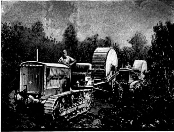
Fig. 3—Transporting cable reels through Allegheny Mountains
