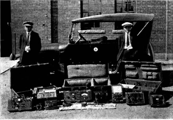
Fig. 10—Illustration of a Typical Transmission Testing Team Layout
