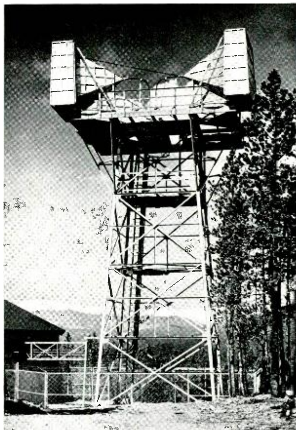
Radio-relay tower atop Buckhorn Mountain in Colorado on the Denver-Oakland relay route; the repeater point amplifies the television signal.
