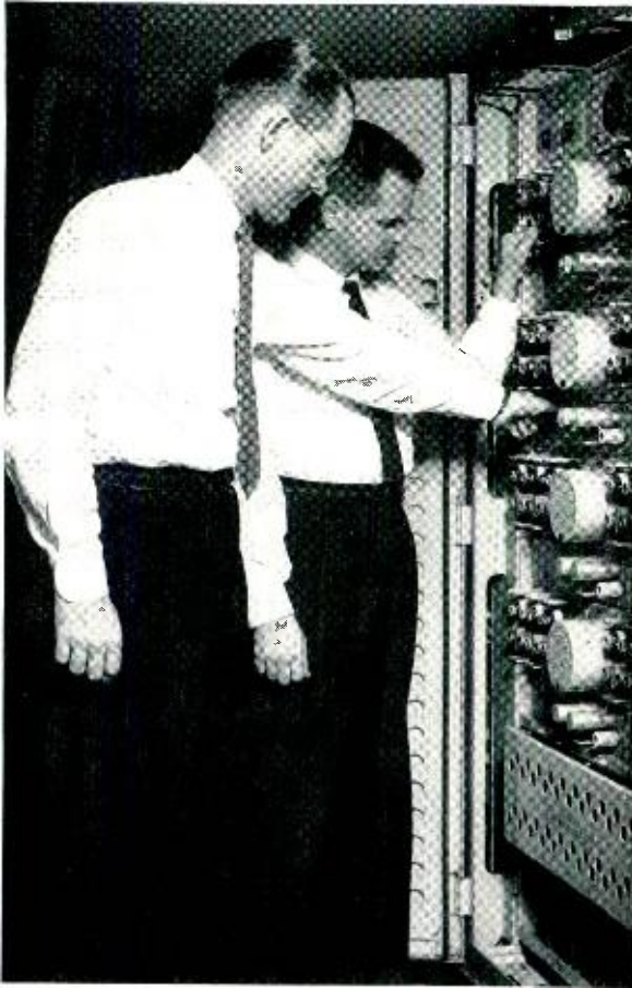
P. L. Hammann, left, and J. L. Troe examine front panel of computer. Panel is mounted on hinges to permit easy access to components in rear.
