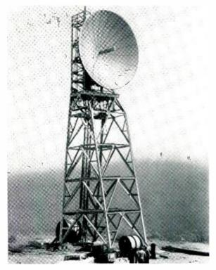
The lateral communication system transmits one thousand watts from 30-foot parabolic antennas.
