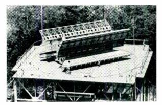
The automatic search radar, shown here before the radome has been erected, uses two antennas of a special design, operated back-to-back.
