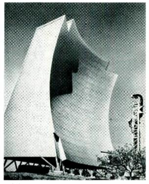
DEW Line terrain sometimes presents difficult or unusual transmission problems. Here, the lateral system uses higher-powered, sixty-foot antennas.
