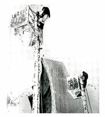
Western Electric installation experts adjusting "side-leg" antennas at White Alice site. These small antennas provide communications to nearby points; large antenna is used for long distances.
