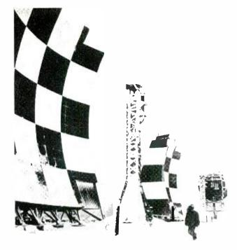
"Beyond-the-horizon" antennas transmit and receive over distances up to 200 miles in the network.
