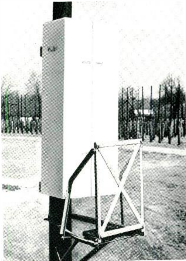
Fig. 4— Model of pole mounting arrangement to be used in the standard system. Concentrator and terminal box are independent of each other but are mounted together.
