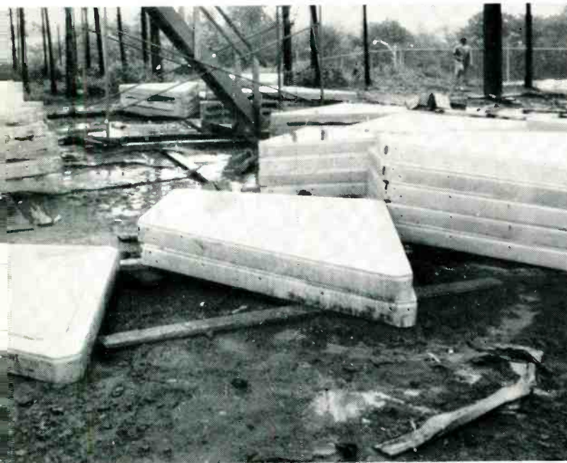
Steps in the construction of geodesic "radome," which has become a symbol of the Arctic DEW Line project.
