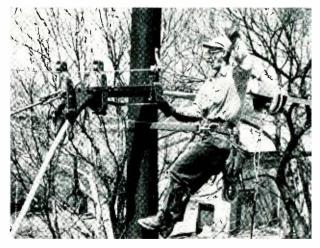
Fig. 4 — The workman, Otto P. Stemler, Jr., New Jersey Bell lineman, signals to halt the tow truck as the clevis passes the pole.
