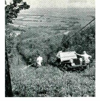
As part of the continuing effort to simplify and economize operating procedures, the Laboratories has investigated chemical control of brush along telephone rights-of-way. Some of the chemicals ordinarily used for weed control also kill the heavier and woodier plants. Extensive field tests indicate that three of these new plantkilling chemicals can do an effective job at lower cost than manual methods.
