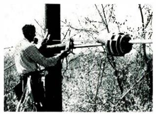
Fig. 3 — Raising the lever lifts the rear arm above the strand when the guide is supported on the front arm and the clevis, permitting the rear arm to be swung toward the workman to clear the pole.
