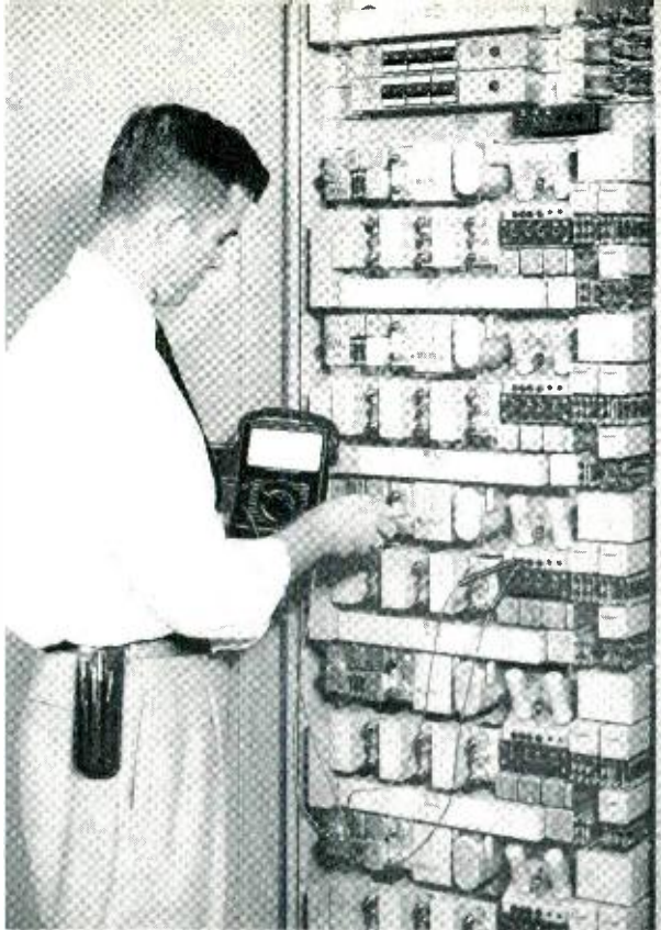
Fig. 2 — G. Plaag of the New York Telephone Company adjusts one of a group of multi-frequency receivers associated with incoming senders.
