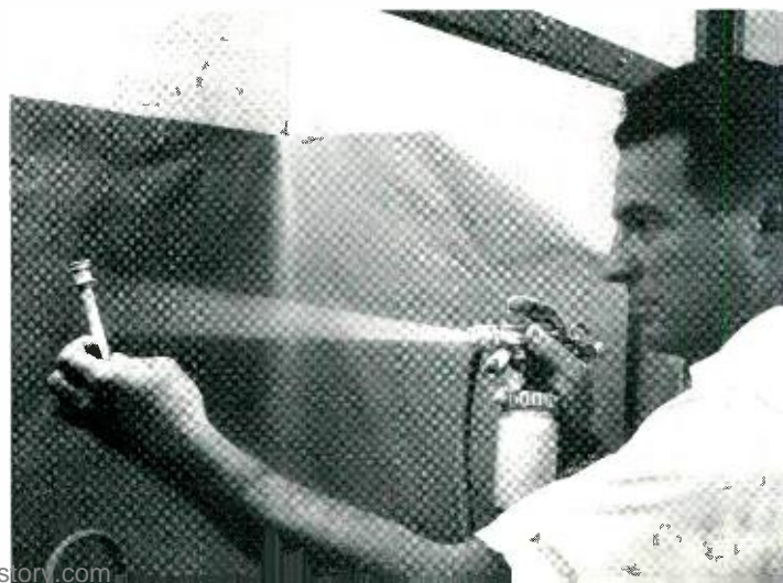
Fig. 2 — N. H. Bagley spraying glaze on a submarine cable component.
