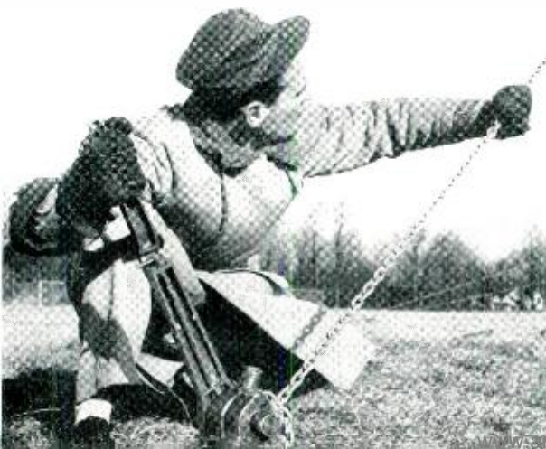
Fig. 4 — R. M. Wheatley operates the chain hoist to raise the antenna into position.
