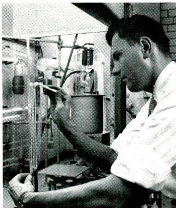
Fig. 2 — J. E. Jamieson installing the tantalum tape upon which silicon will be deposited during the reduction process.
