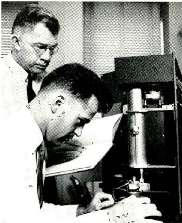
Fig. 7 — P. A. Byrnes (right) moves germanium specimen with respect to beam of light while G. P. Carey plots data for lifetime measurement.
