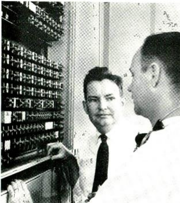
Fig. 1—The author (left) and J. M. Repholz, switchman, New York Telephone Company, discuss a sender under test by the test circuit, New York City CMA installation.
