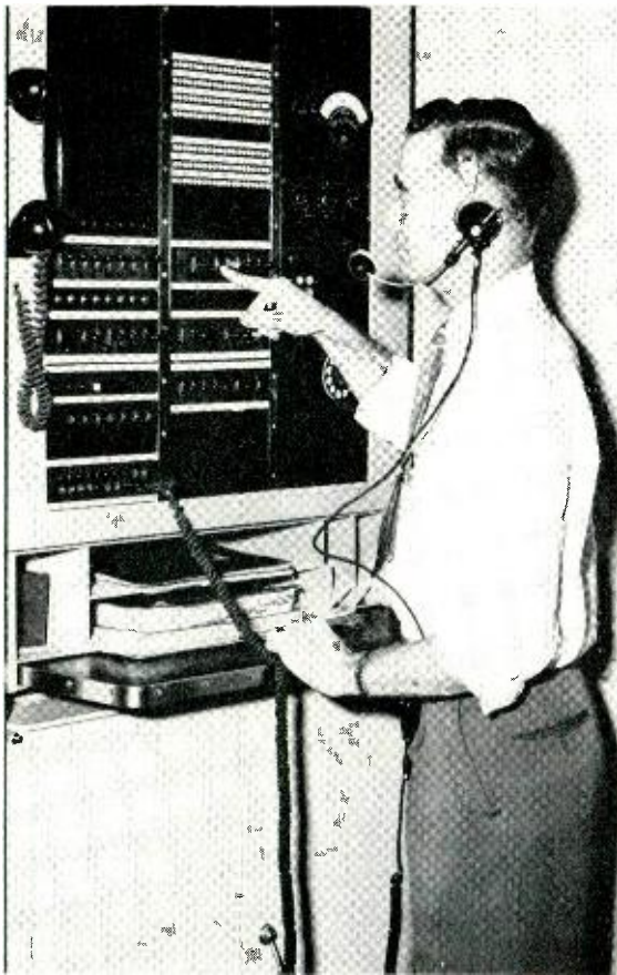
Fig. 1—W. D. Frietsche, New York Long Lines, starting a test cycle at the automatic outgoing intertoll trunk-test circuit test panel.
