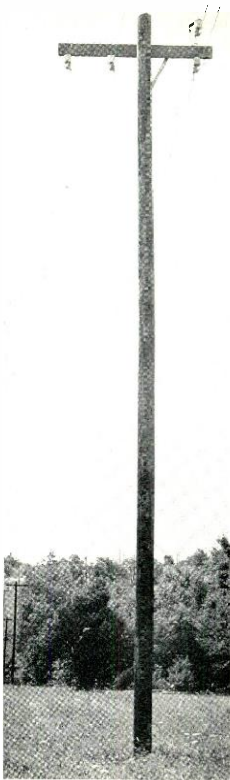
Fig. 3 — A complete ground-erected two-pair line, showing horizontal and vertical mountings of suspension insulators.
