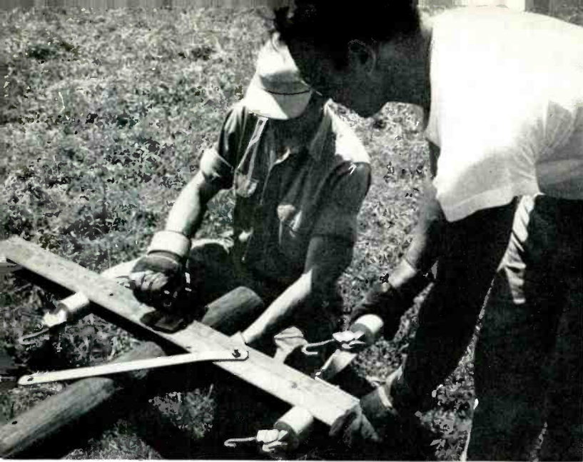
Fig. 1 — Prior to erection, the pole and all of its fittings are being assembled on the ground by J. D. Apgar (left) and V. P. DiLullo of the Chester Laboratories.
