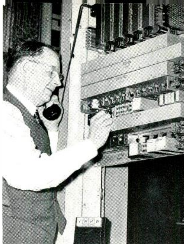
Fig. 2 — Francis B. McKeon of the New England Company makes a routine test on "Bells and Lights" central office equipment.
