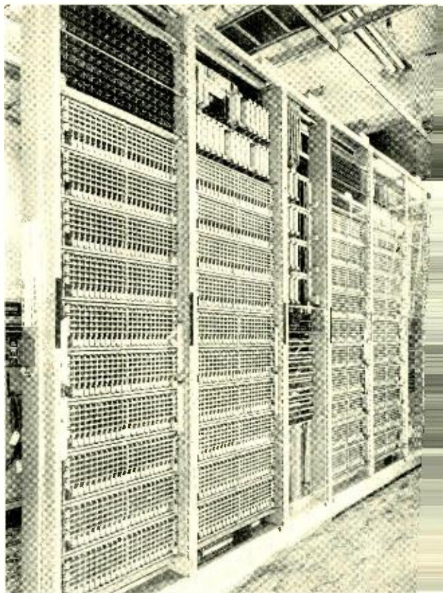
In establishing telephone connections, the crossbar switching system processes information.
