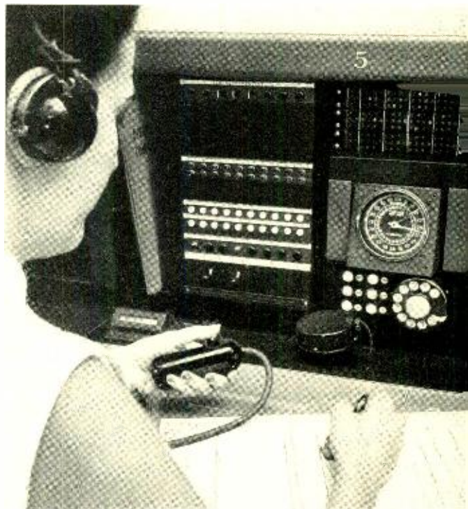
Fig. 5 – Closeup of a No. 12 service observing position.
