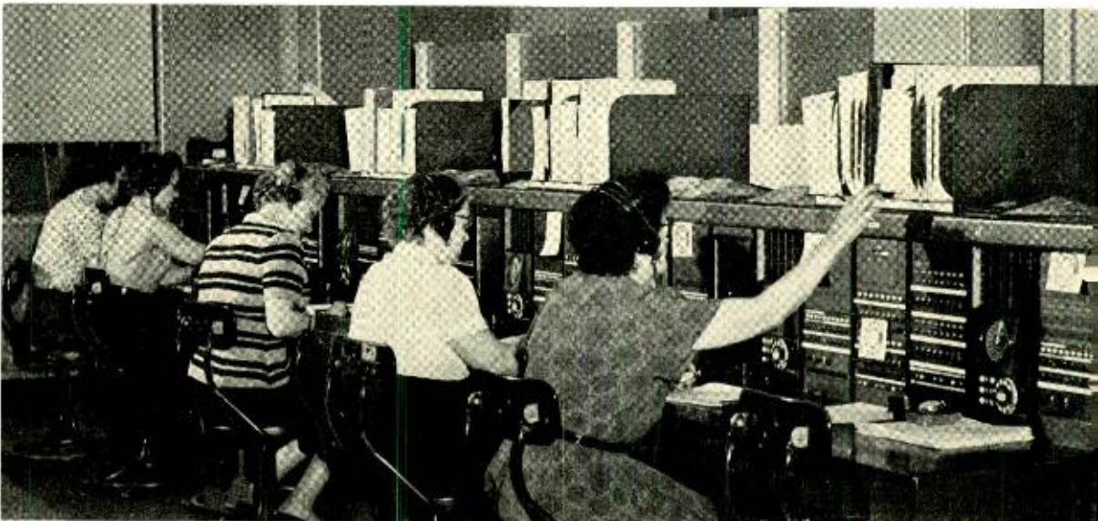
Fig. 1 — Four sections of a No. 12 service observing desk at the 36th Street Building in New York City.
