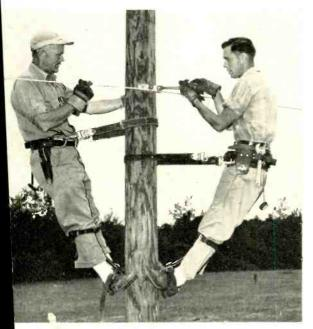
Aloft, the cushion body belt provides a soft cushion about the hips, preventing chafing or abrasions possible under extreme weather conditions or during long working periods. The man at the left wears the body belt normally provided.
