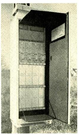
Fig. 2 - A pole-type repeater cabinet equipped with four repeaters.
