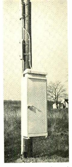
Fig. 3 - A repeater mounted on a stub pole on an underground cable route.
