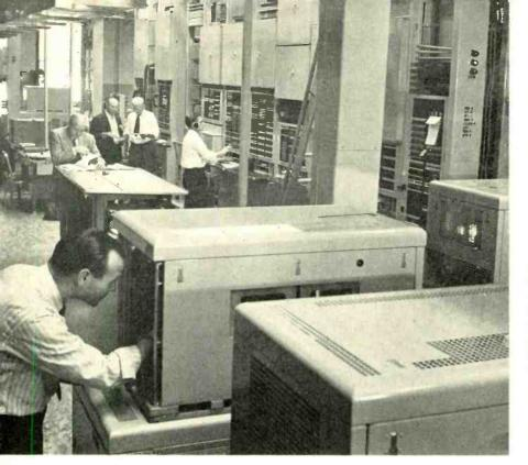
Fig. 3–Part of a 4A sectional center showing a group of card translators in the foreground and another in the background (left) with the maintenance center between them.
