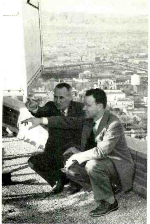
J. H. Miller (right), field engineer at Denver, with Neil Mills, Long Lines Equipment Maintenance Supervisor, examine the exterior cover of the antenna for the microwave radio relay station atop The Mountain States Telephone and Telegraph Company building in Denver.
