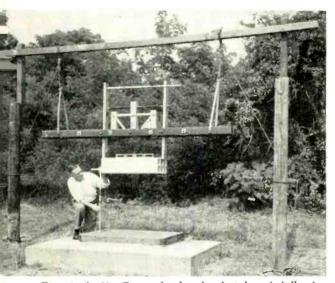
Fig. 1–J. H. Gray checks the height of fall of a six-duct conduit after it has been carefully leveled.
