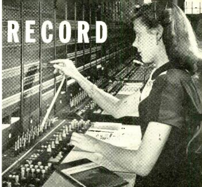
Fig. 1—A position at a No. 5 switchboard used with the A4A system for handling delayed calls.
