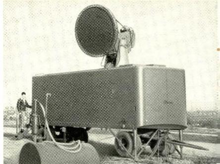
The new fire-control radar and the van in which it is transported.
