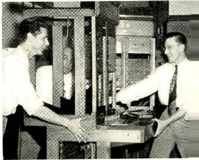
Rearranging of the PBX board in the telephone exchange at West Street to concentrate more lines per position accordance with New York Telephone Company practices, Thomas Condon, at the left, is shown disconnecting position. Dismantling a position, are left to right, Thomas Condon, James Sharp and William Walter.
