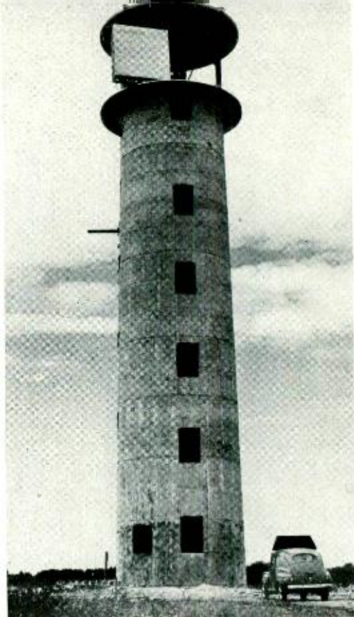
This radio relay tower, on the Bell System television networks between Chicago and Milwaukee, is at Lake Zurich, Ill.
