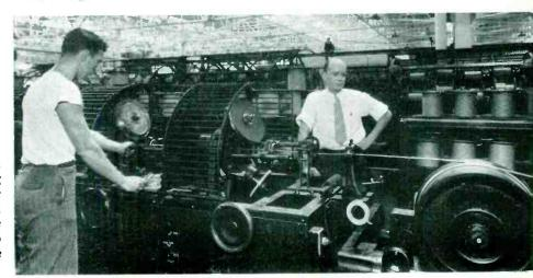
Fig. 5 – Application of copper shielding tapes to a video pair is observed by R. B. Ramsey as the operator prepares to change a pad of the tape
