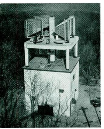
Fig. 2-One of the repeater stations of the New York-Boston system showing antennas on the roof
