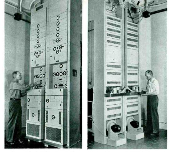
Fig. 4-Front (left) and rear views of two relay bays at a repeater station
