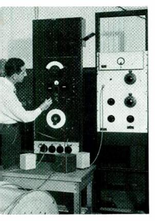
Fig. 1-G. J. Schaible at the Point Breeze Works of the Western Electric Company measures insertion loss on an experimental length of video pair used for television pick-up installations
