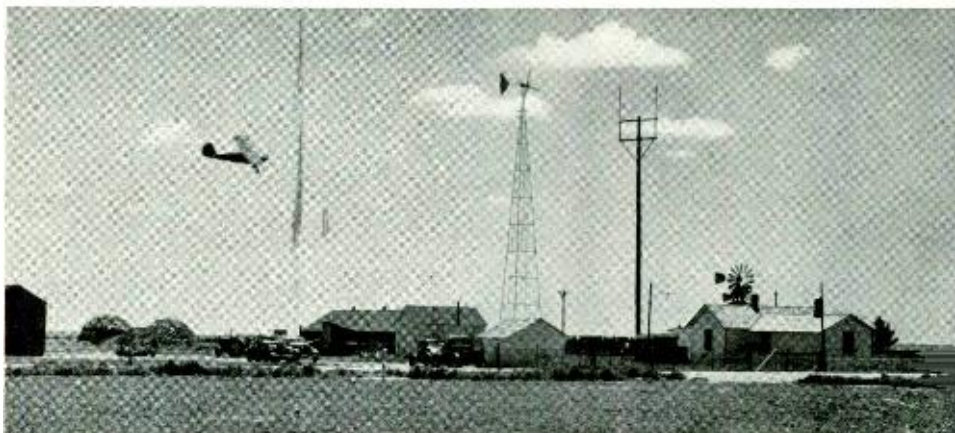
C. F. Blackwelder's ranch receives radio telephone service through the two antennas on the pole to the right of the windmill, which is used for power generation. Mr. Blackwelder is shown approaching in his private plane
