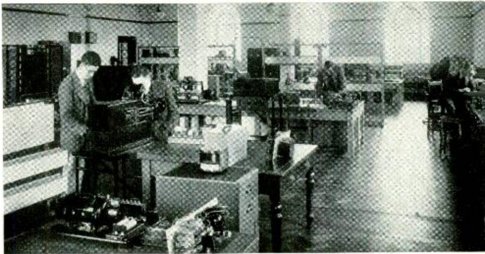
Fig. 2—Laboratory devoted to the development of central-office switching systems
