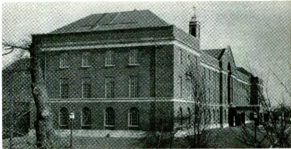
Main research building of the British General Post Office
