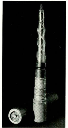
A section of German coaxial cable, showing elaborate use of styroflex insulation to suspend the central conductor in the pipe
