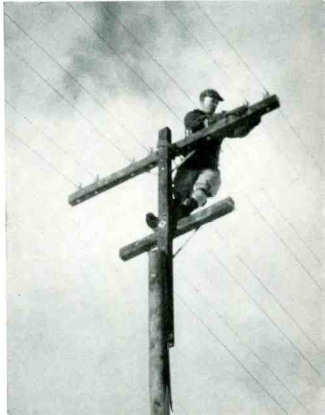
Fig. 2—The crossarms also serve as side arms and pole-top extensions. A half-length arm can be used as a foot support for the lineman
