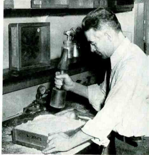
He rams the sand mix and then smooths and finishes the core
