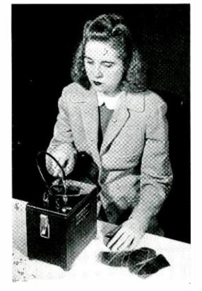
Fig. 5—The spark test locates conducting regions in block mica, and permits defective material to be rejected before applying the classification test
