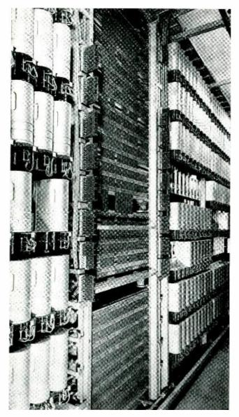
**MPROVED** graded-multiple trunking arrangements have recently been made available for standard step-by-step offices which result in material economies in selectors and other equipment, and very substantially reduce the cost of making periodic revisions in the number of graded multiple trunks in existing offices.
