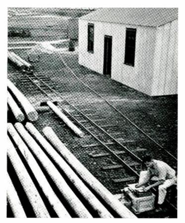
Fig. 1—Measuring the resistance of untreated southern pine telephone poles with the Laboratories' electrical apparatus for determining the moisture content of timber. A. H. Hearn is shown making tests at a creosoting plant in South Carolina
