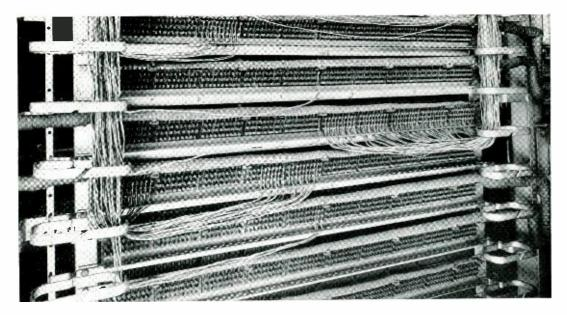
Fig. 8—Rear view of DTA frame showing cable forms coming from the selector banks and the iumper cross-connections going to the terminal strips for the trunks to succeeding circuits
