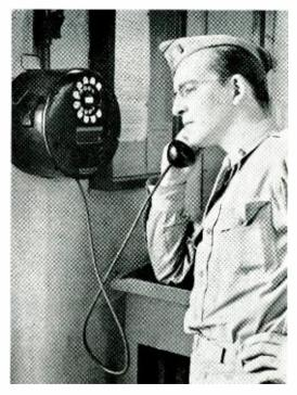
Explosion-proof telephone used in the communications system of a TNT plant
