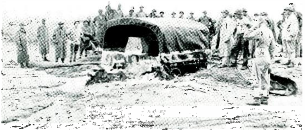
After some of the mud was dug away, tow lines were attached and the trailer with its Electrical Director was hauled out of the mud hole
