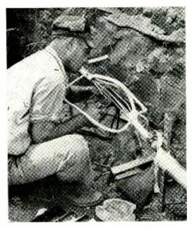
Splicing a coaxial cable now being laid between Atlanta and Jacksonville
