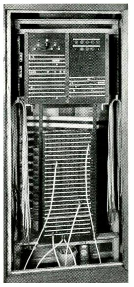
Fig. 2—Traffic supervisory panel used in connection with the handling of delayed calls in the crossbar toll system
