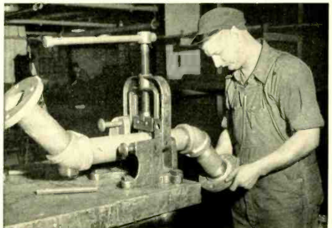
Teddy Olsen of the Building Shop makes up a pipe detail for a cooling system
