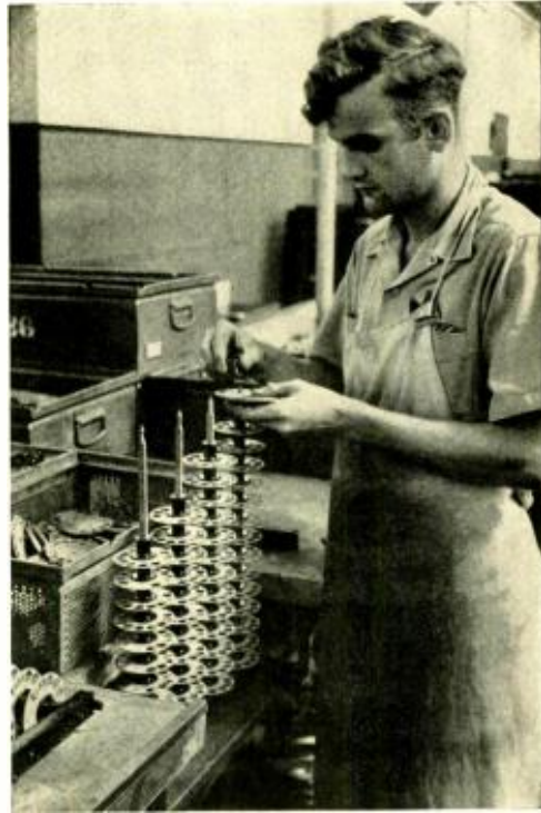
Steel is now being used for the manufacture of the telephone dial finger wheels in place of aluminum, a vital defense material
