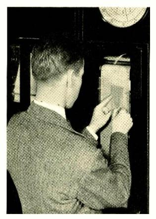
TO KEEP a continuous check on the relative rates of the crystal clocks which comprise the Bell Laboratories' frequency standard, and also of their absolute rates in terms of radio time signals, a spark chronograph is used. It permits a continuous intercomparison of the timekeepers by automatically recording on a slowly moving chart a curve for each clock. These curves indicate at any point the difference in time between the clocks.
