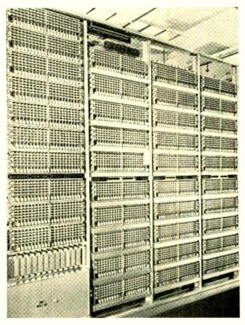
Fig. 1—A line-link bay at the Troy Avenue Office, which employs three bays of primary switches
