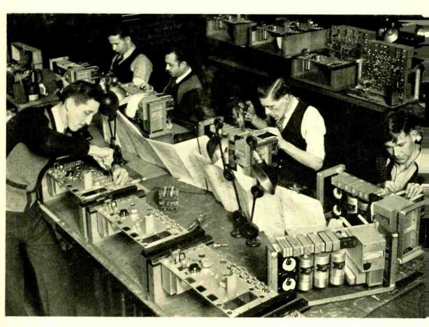
2B Regulators are assembled and wired at the Kearny works of the Western Electric Company. The characteristic curves below show (a) varia-
