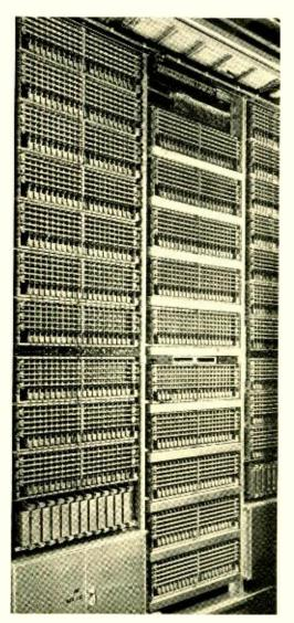
N the step-by-step and panel systems each subscriber line is brought to two switching frames. One of these, the line finder, is used when the subscriber is placing a call; the other, generally known as the final frame, is used when a call is being completed to the subscriber. The crossbar system differs radically from these earlier systems in this respect, since with it a subscriber line is connected to only one frame—the line link—which is used for both originating and termi-266
