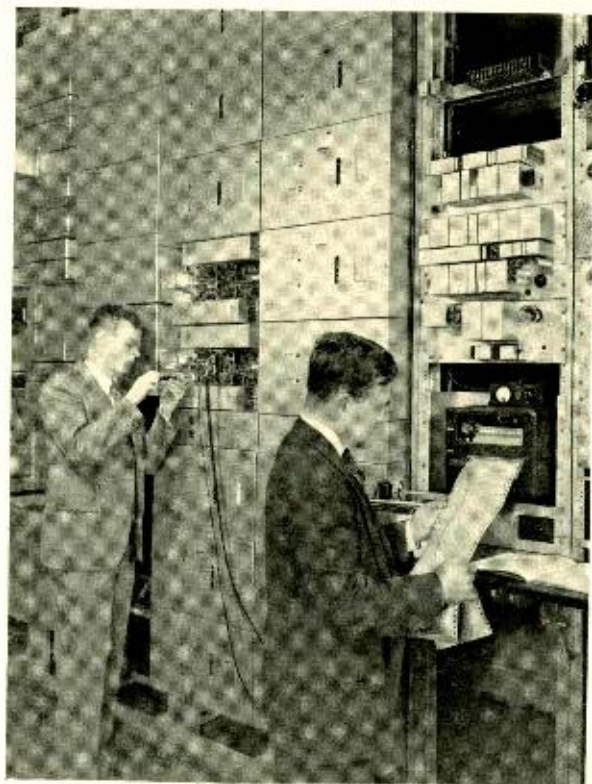
Fig. 2—Installation of channel equipment located at 32 Sixth Avenue, New York
