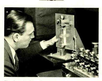
The volume of carbon used in a handset transmitter being measured by A. P. Besier of the Telephone Transmitter Laboratory
