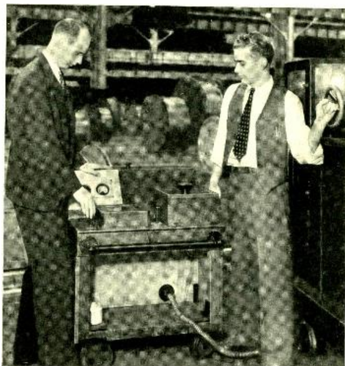
Direct-current breakdown test being applied to sections of the coaxial cable during manufacture by A. S. Windeler (left) of the Laboratories' Point Breeze staff and J. Brown of the Western Electric Company. (See page 325)
