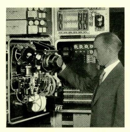
V. E. Rosene of the Systems Development Department displays the inner mechanism of the pilot-wire controller used for transmission twist regulation on cable-carrier telephone circuits. This equipment corrects for the change in attenuation in a frequency band caused by temperature variations of the cable. An associated equalizer switch box is shown above the controller
