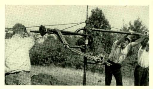
Fig. 6—Earth anchors of the screw type used in guying poles in sand and swamp land are tested by measuring the torque required to force them into the ground
