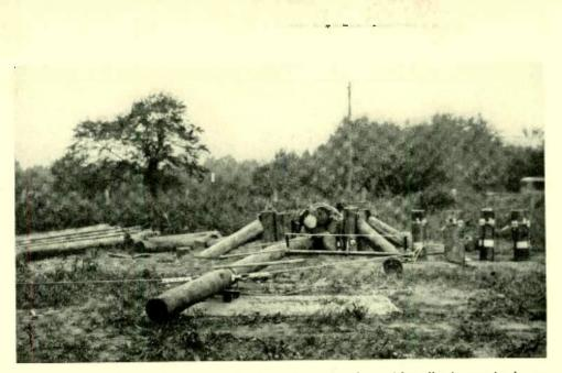
Fig. 5—Sidewalk guy fixtures, used where clearance above sidewalks is required, are tested at the Chester field laboratory by mounting them on poles supported horizontally close to the ground for convenience of measurement
