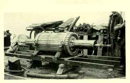
Fig. 5-The new submarine loading coil case ready for installation
