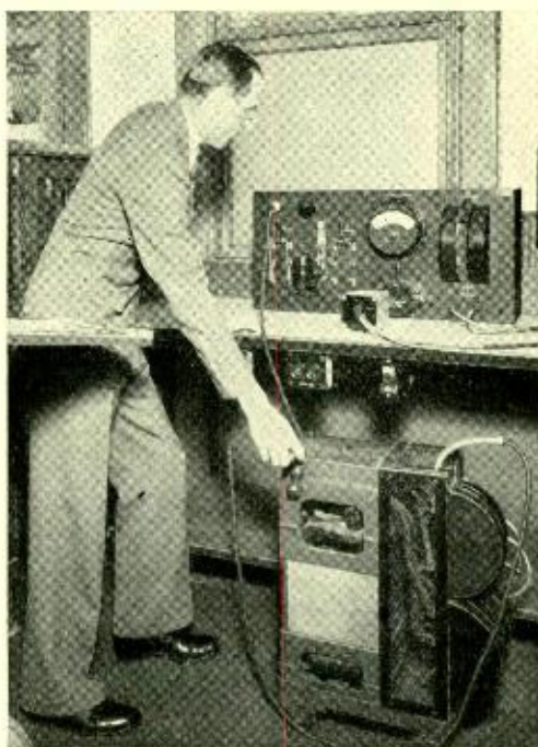
Fig. 8—J. P. Whistler operating the induced voltage testing set
