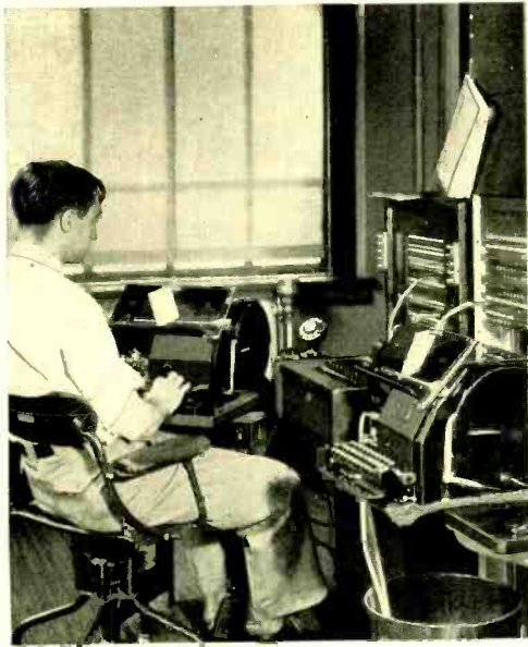
Fig. 3—A 65B1 teletypewriter board installed in Denver, Colorado
