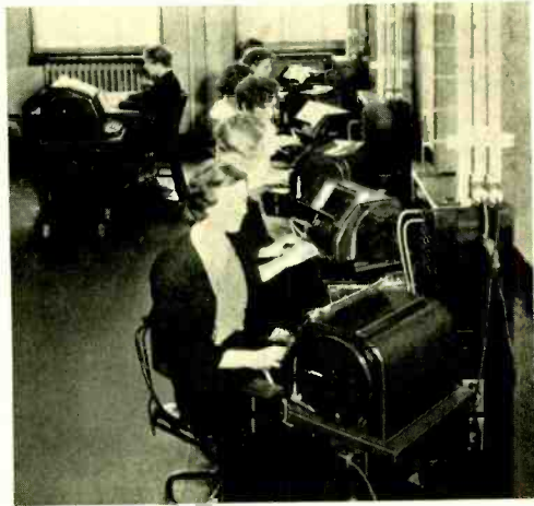
Fig. 4—An installation of the No. 3 teletypewriter switchboard in Akron, Ohio
