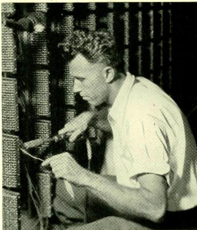
Fig. 3—Millions of soldered contacts are an important element in the Bell System plant
