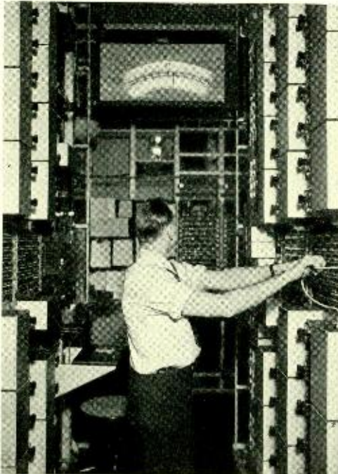
Fig. 1—A trial installation of the projection metering equipment
