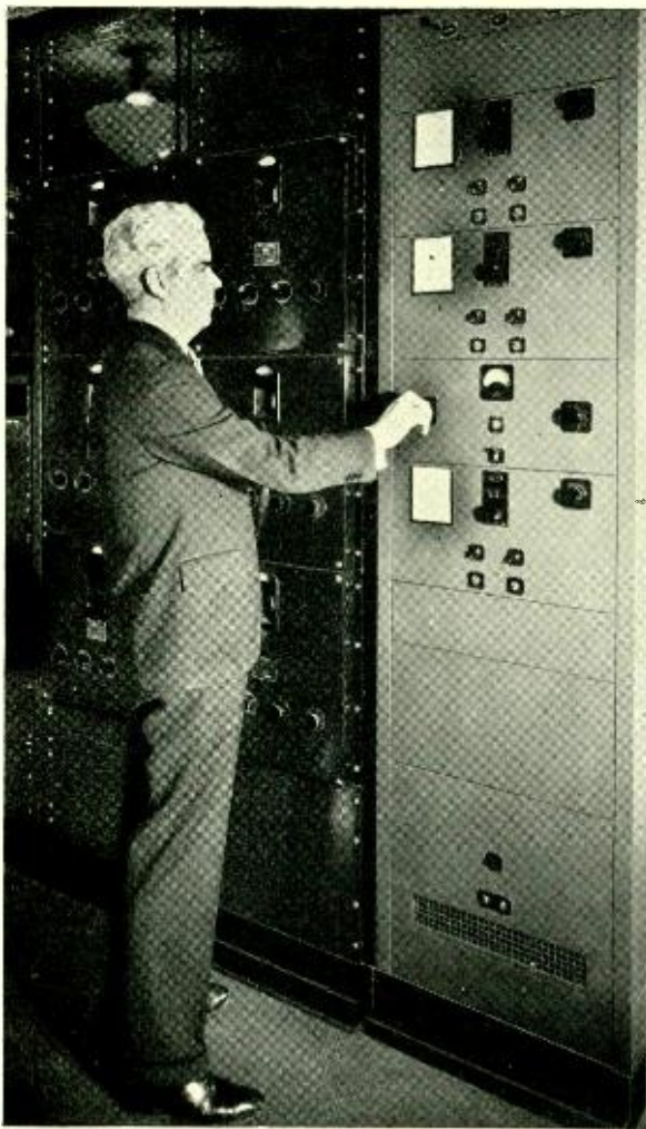
Fig. 1—H. R. Martin, Superintendent of Communication at the Waldorf, tunes the short-wave receiving unit
