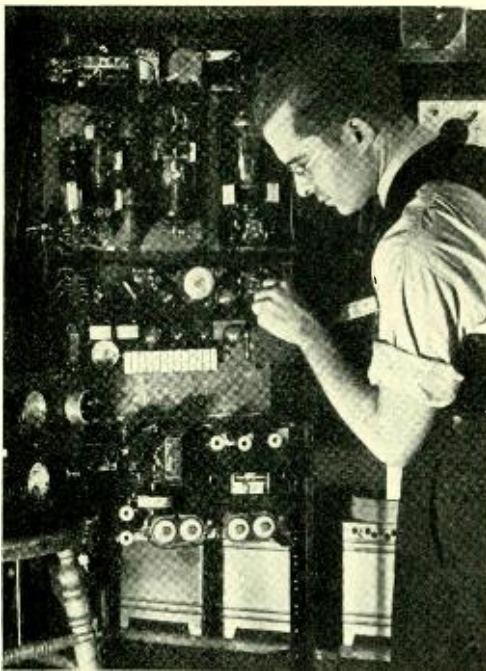
Fig. 6—R. R. Blair with experimental repeater and automatic control circuits
