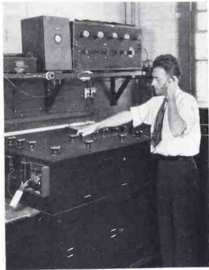
Fig. 3—J. A. Kater making a capacity measurement on a 141-A condenser
