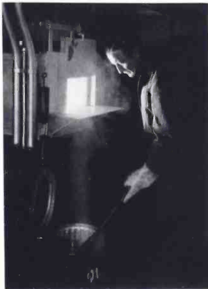
Fig. 6—Heat treating has a pronounced effect on magnetic properties. I. H. Hirten is here shown quenching a test specimen
